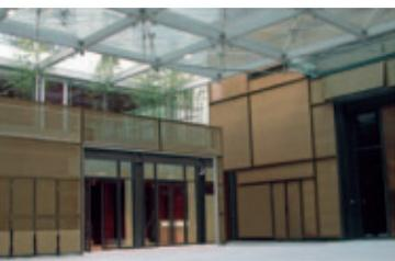
*A subtle suggestion of wings was recreated using nets in copper alloy with angles of the same material, acting together as a unique sun shade.*
